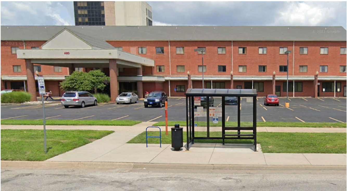
Figure 3-4: Bus Stop on Westbound 6th at Jefferson showing shelter (Source: Google)
